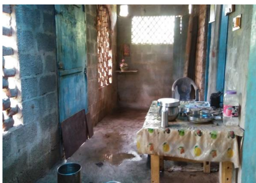
Leaking roof and damp floor- Raveendran () Ward 8
