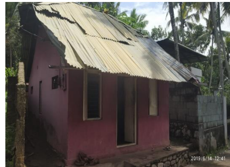
Dilapidated Tin Roof- Shylaja (166558) -Ward - 10
